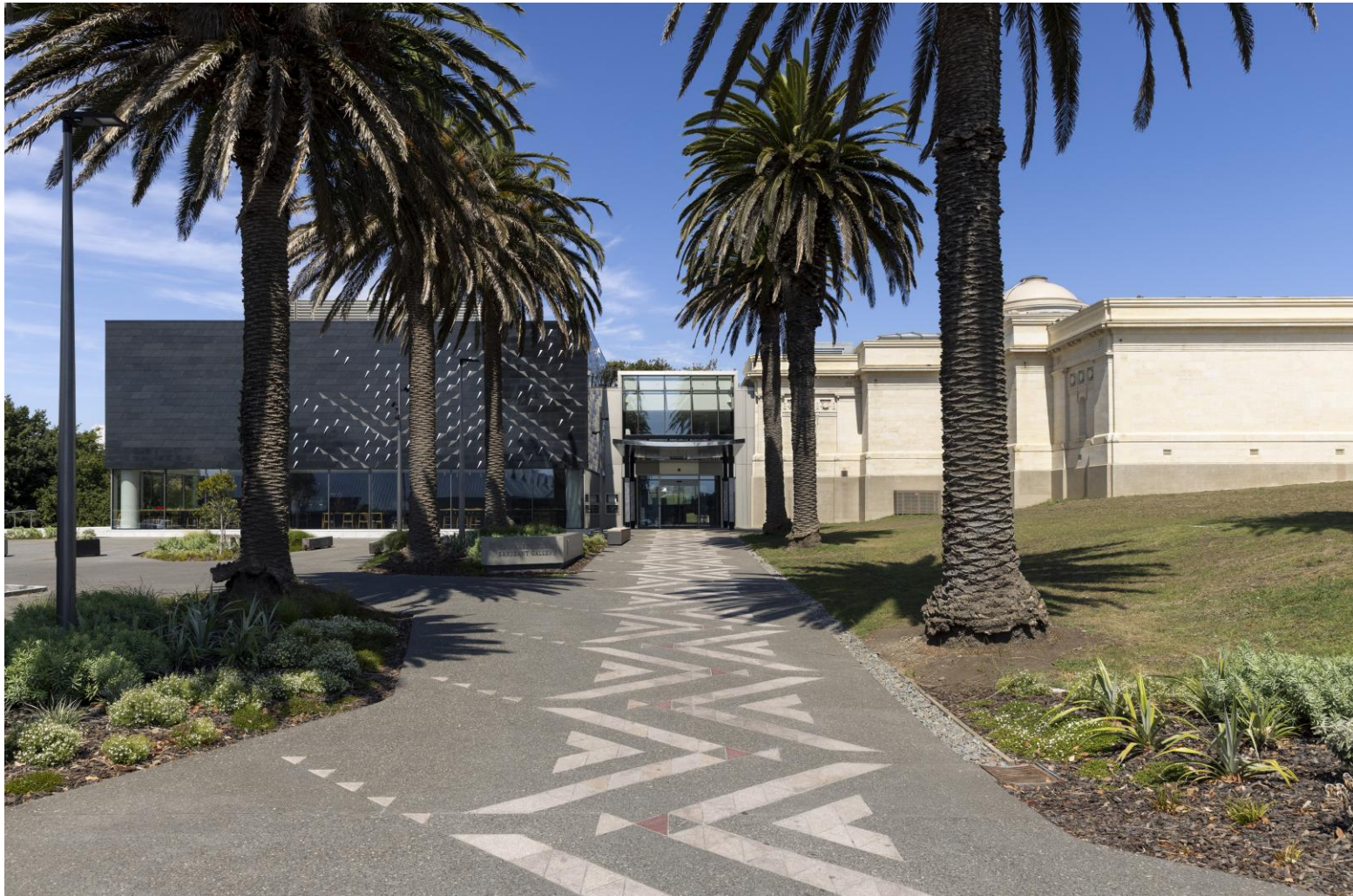
Figure 2.1 Sarjeant Gallery new entrance at the north end of the original building.
