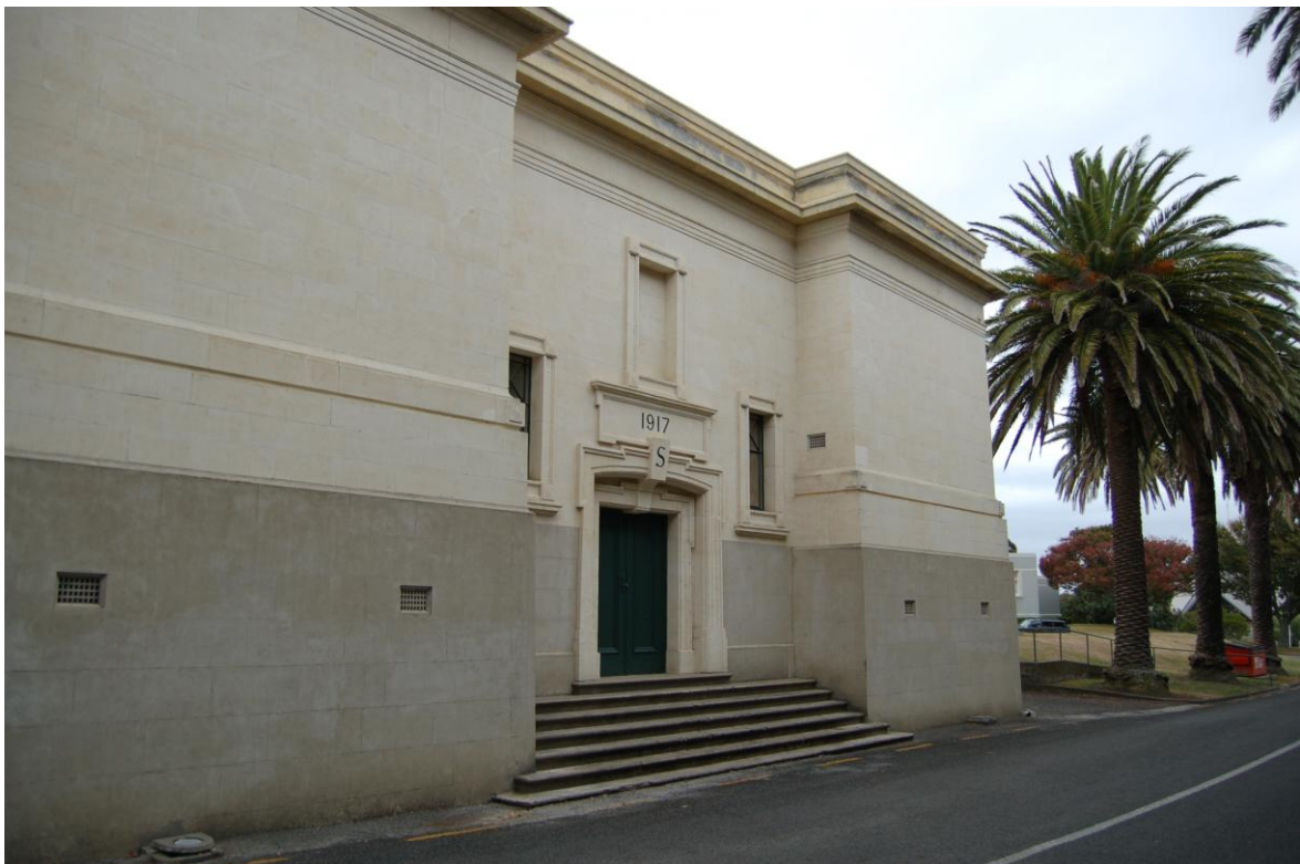
Figure 2: Northern Elevation: Entrance at basement or road level (closed in 2014) (This entrance was lifted in the redevelopment to be at the gallery level, with the architectural features retained and a new link bridge installed connecting the old and the new buildings)
