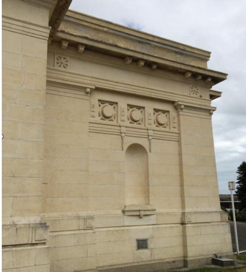
Figure 5: Architectural features at West Wall (closed in 2014)
