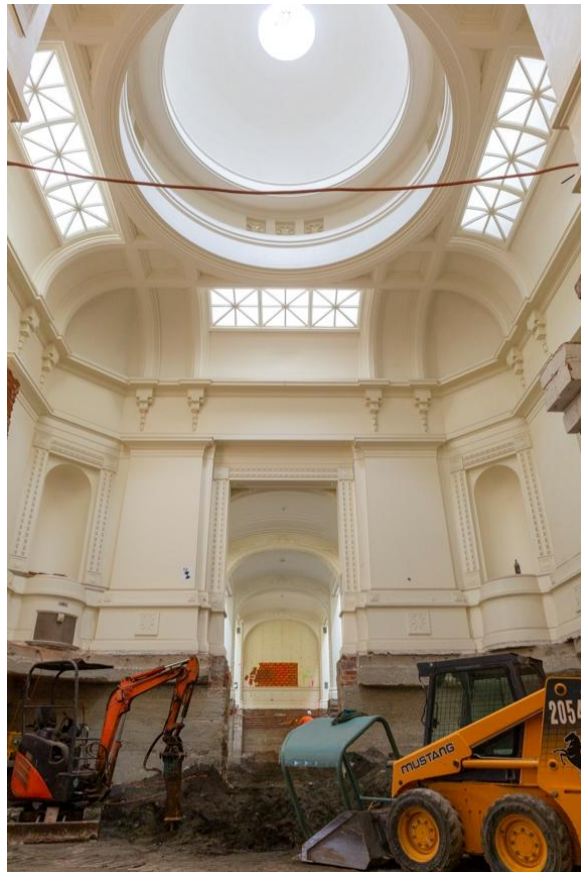
Figure 1.3 Excavation in progress – Core area.
