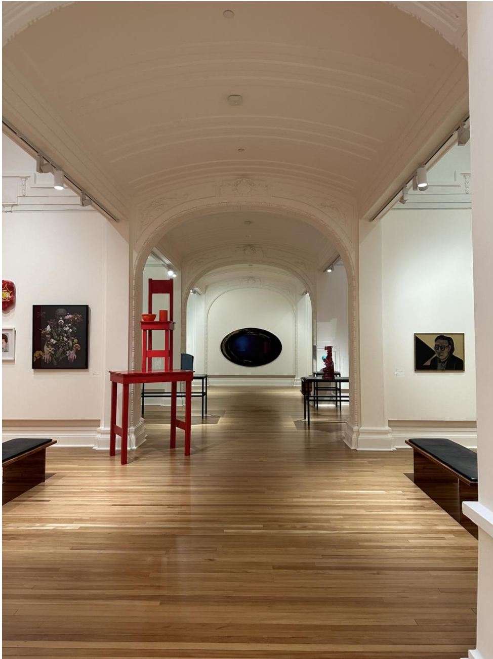
Figure 2.5 View of the interior with the original timber floor boards reinstated and laid over the new concrete floor.
