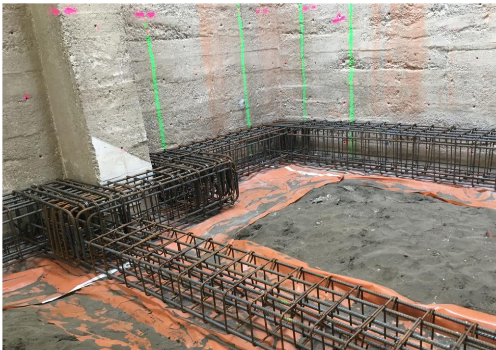
Figure 1.4 Ground beam reinforcing installed, wall starters to be placed.
