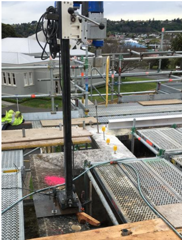
Figure 1.7 Drilling of holes for a prestress bar at roof parapet.
