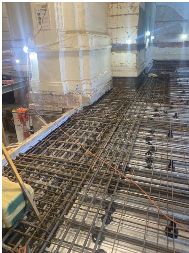
Figure 1.6 Floor slab reinforcing placed.
