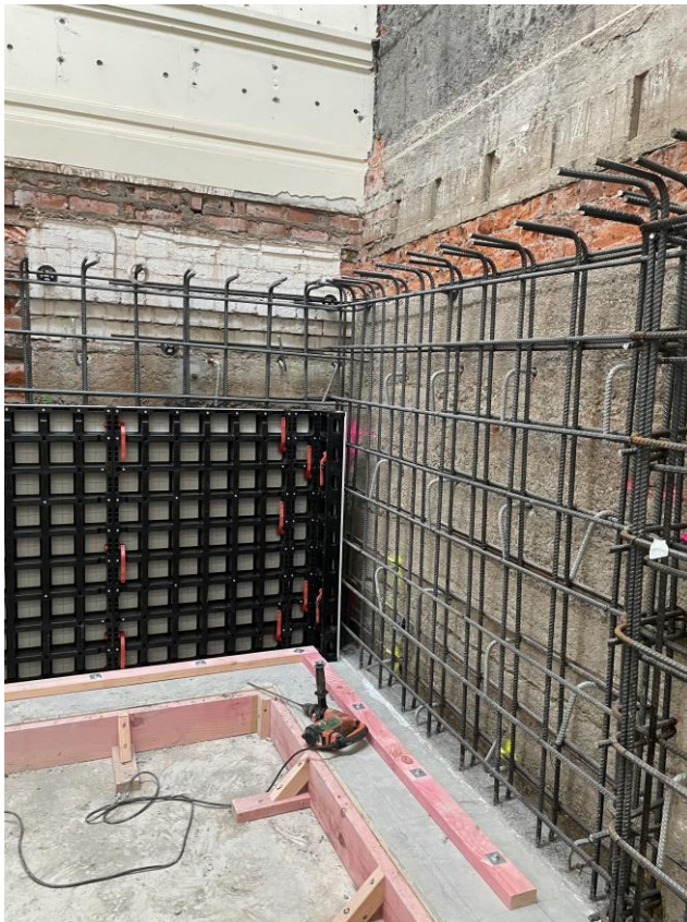
Figure 1.5 Foundation wall reinforcing placed.
