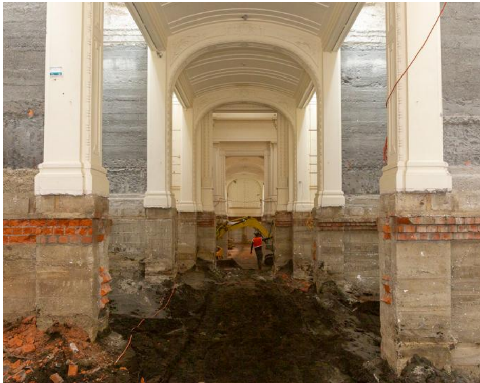
Figure 1.1 Excavation in progress – timber floor removed.
