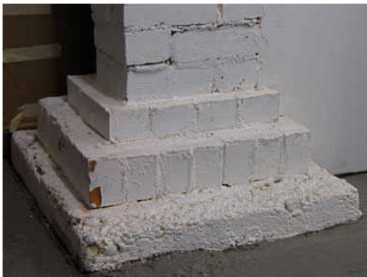
Brick piers standing on concrete foundation.
