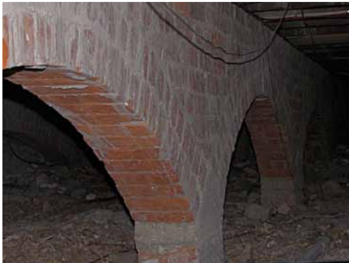
Brick arches in the basement.
