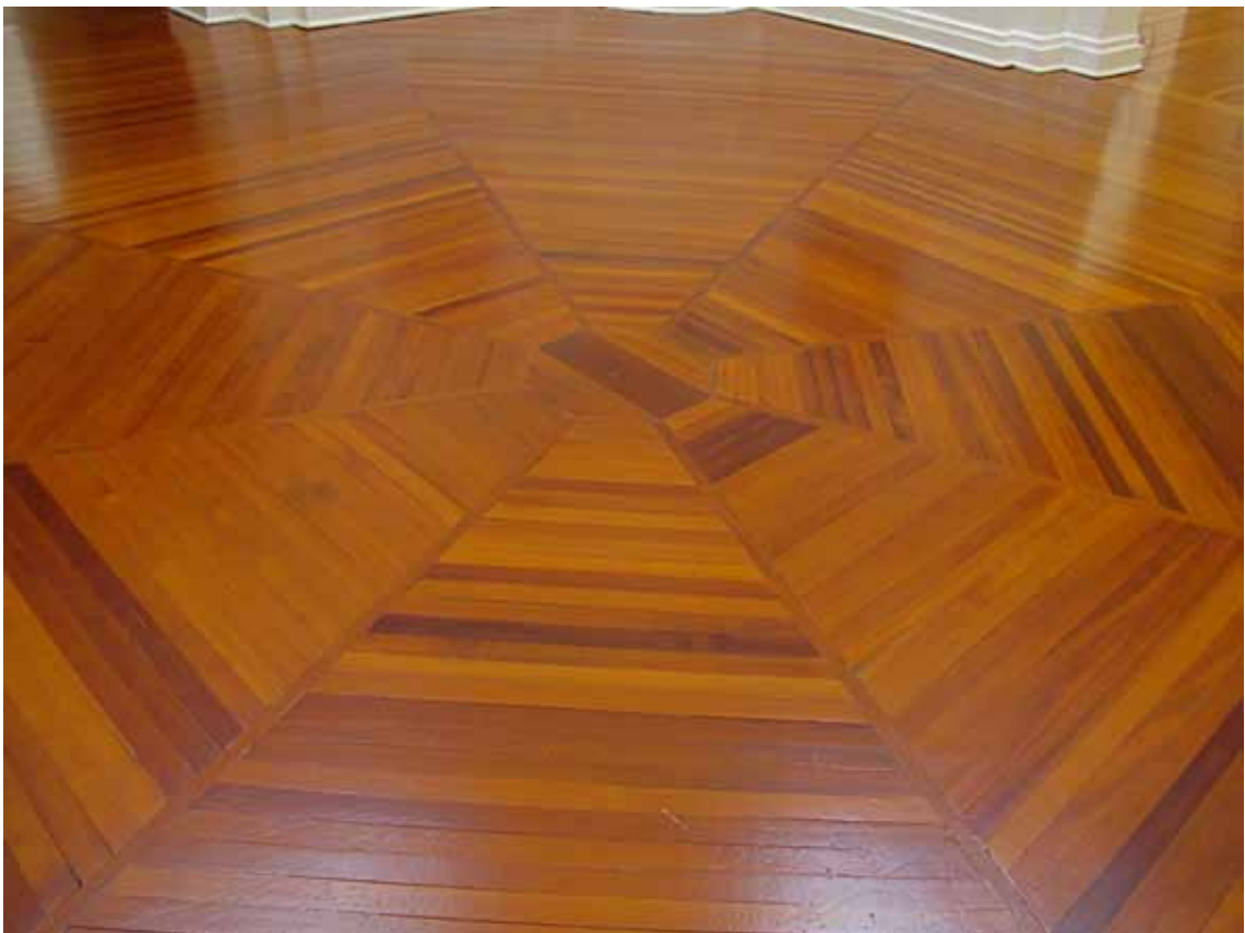
Detail of tongue and groove matai flooring, secret nailed, in the Dome Gallery.
